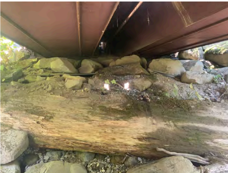
Left Bank Abutment when facing downstream
