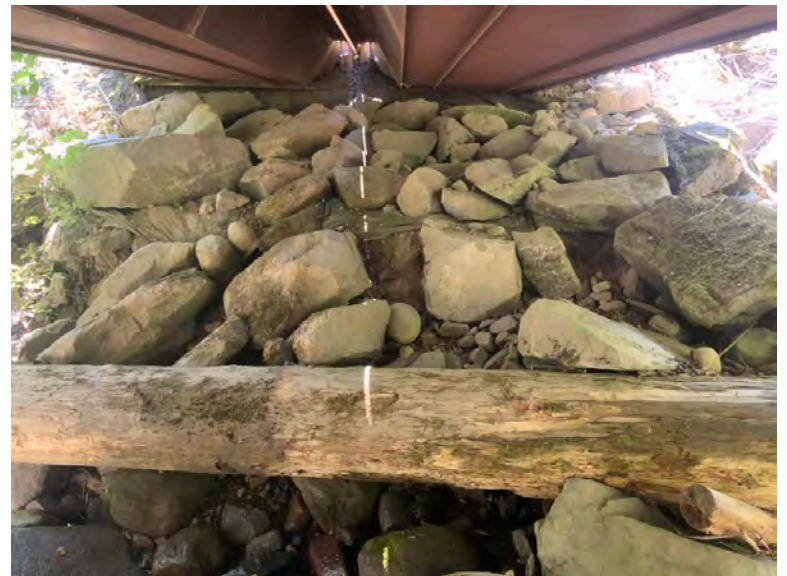
Right Bank Abutment when facing downstream
