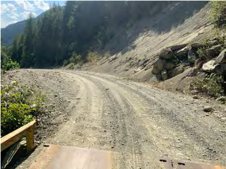
Approach from Right Bank when facing downstream
